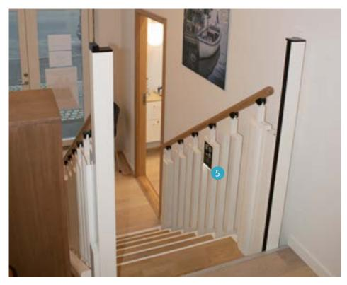
The white staircase with steps covered with the same wood cladding as the rest of the floor, makes the solution appear light and elegant. The FlexStep function both as an ordinary staircase and as a wheelchair lift ensuring people with walking difficulties and wheelchair users to get around safely, even though the clinic has several levels.
