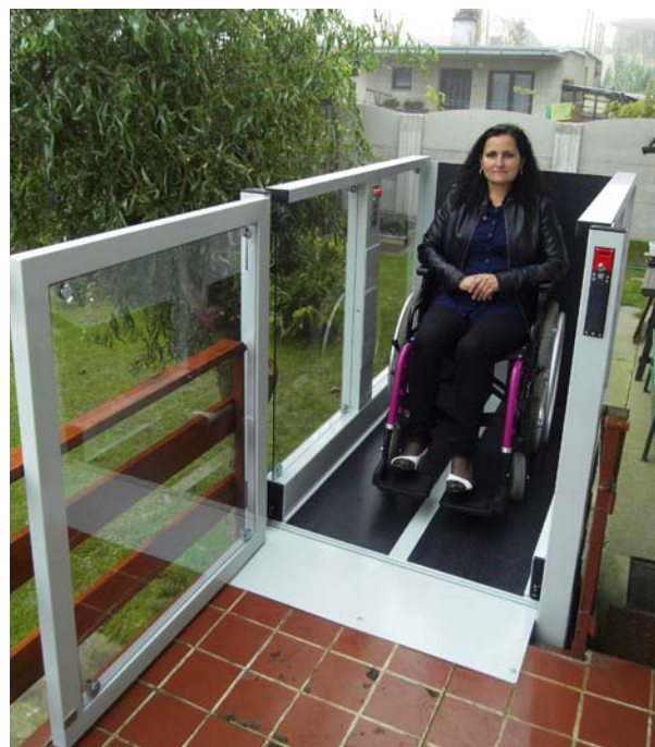
Upper gate and side walls with glass inserts
